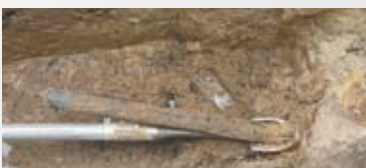
Exchange of ground cables with wash-over method (only at TT)
