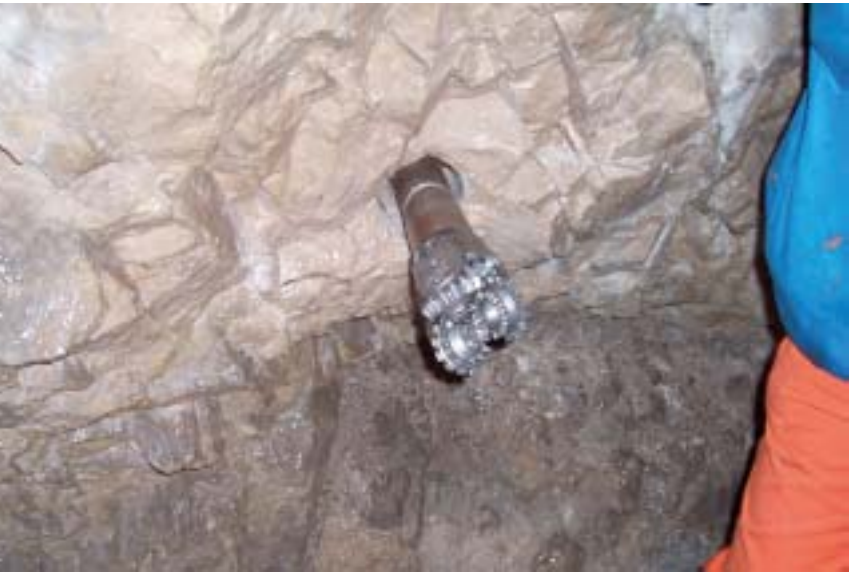
Spot bore up to 150 mm
