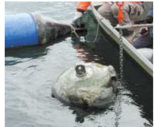
The pontoons which were necessary to hold the pipe string above water in stable position.
