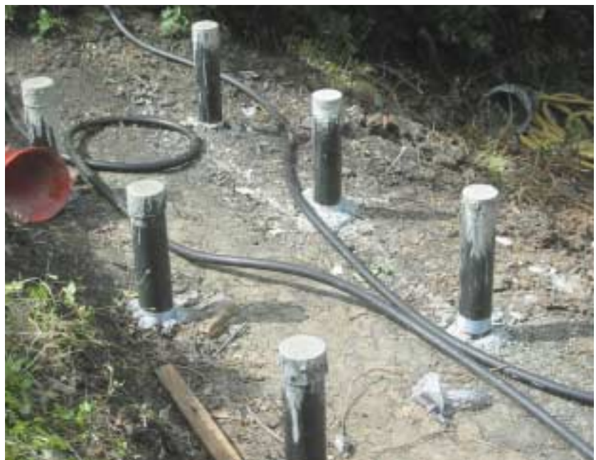
Reinforced concrete piles now firmly in place
