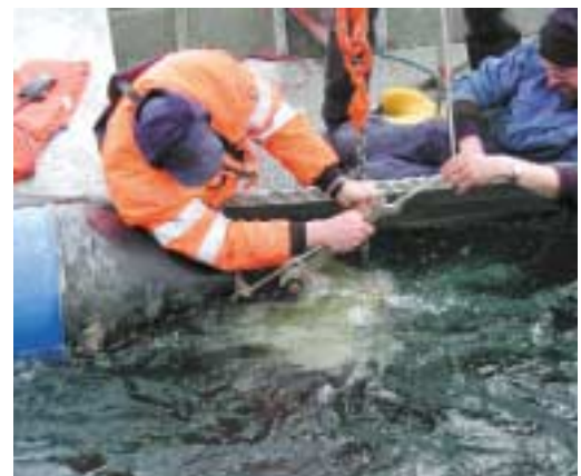
The loaded pipe string with the swimming bodies is pushed into the lake with the help of a cable dredger. Then it is connected to the backreamer.
