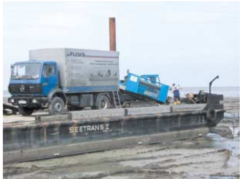
The pontoon carrying the boring equipment.
