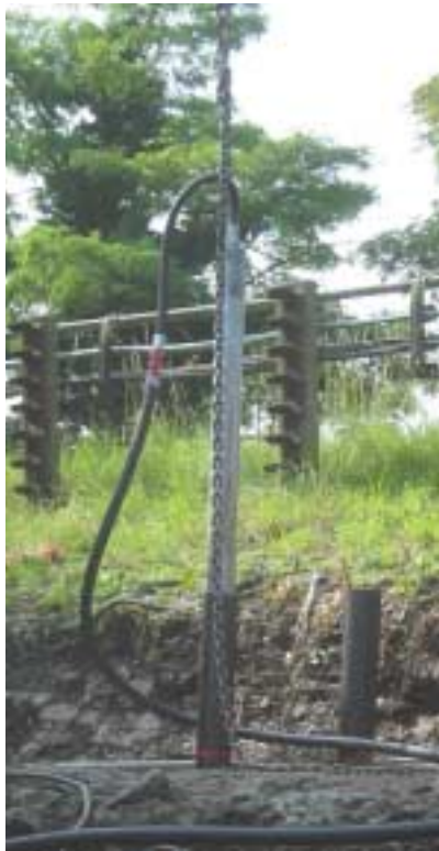
GRUNDOMAT being removed from the pile
