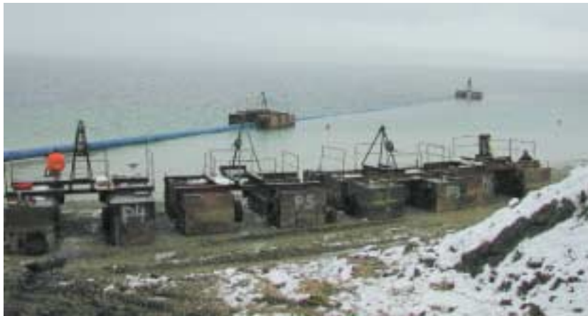
The pontoons which were necessary to hold the pipe string above water in stable position.
