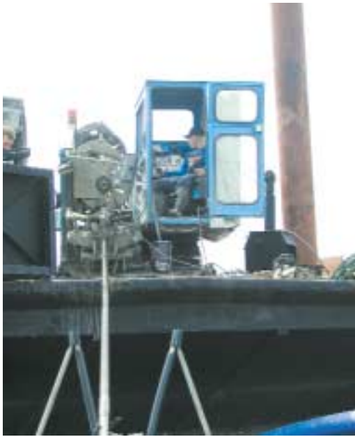
The Grundodrill 12 G-bore unit during the pipe installation
