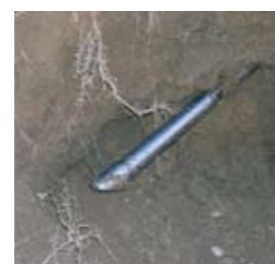
Location of the bore head, arrival and pipe pulling.
