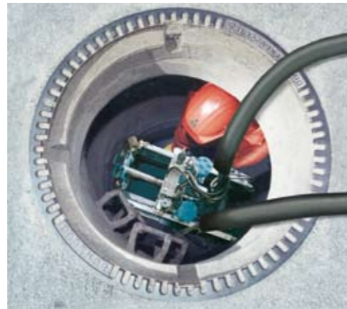
Start from the manhole to the service room of the building
