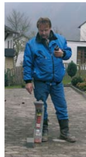
Location of the bore head, arrival and pipe pulling.
