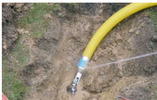
You can pull in single pipes or pipe bundles
