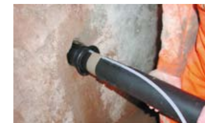
6. Mounting the wall lead-through
