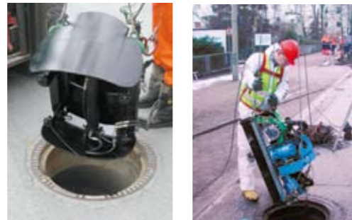
Setting up the working platform and the Grundopit-Manhole
