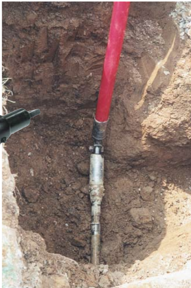
You can pull in single pipes or pipe bundles
