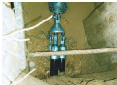
You can pull in single pipes or pipe bundles
