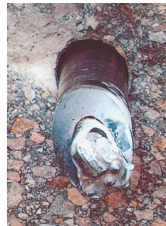
The hammer bore head boring through a concrete wall
