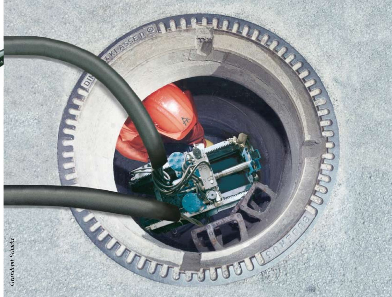
GRUNDOBORE - Auger boring systems pilot steered, e. g. for gradient pipes Model 200S and 400
