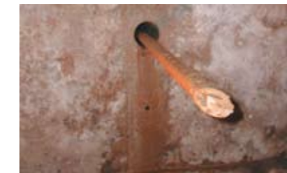
4. "Driving in" the bore head into the cellar
