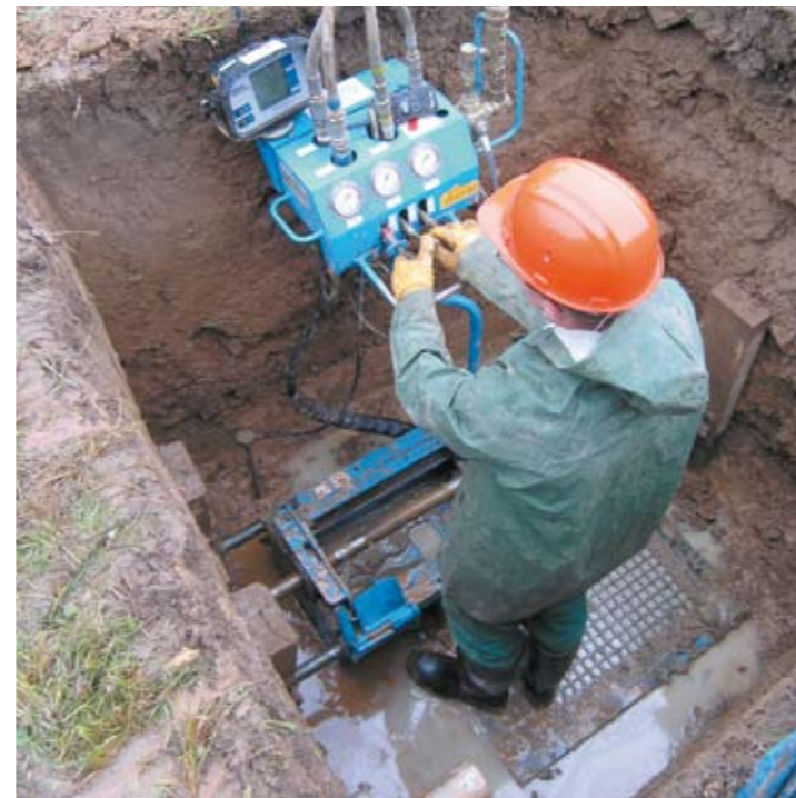
Location of the bore head, arrival and pipe pulling.
