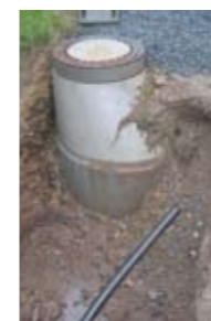
Connection to the sewer network
