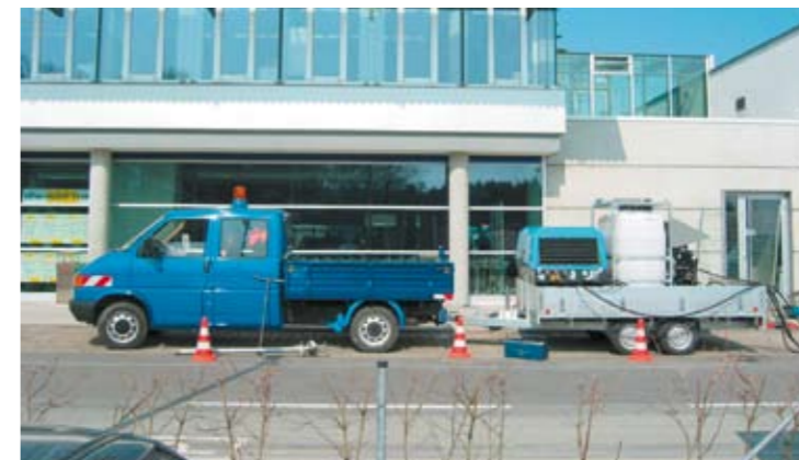
Transport of the boring equipment
