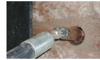
5. Tool exchange / pipe pulling
