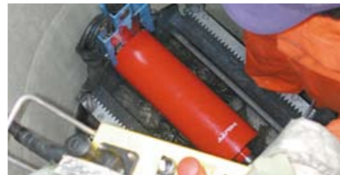
The Grundopit establishing the core hole bore from out of a gully hole. Operation with KA 38.
