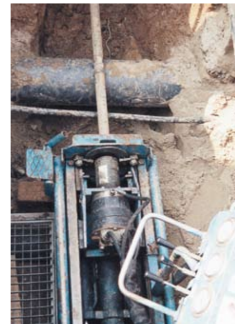
The hammer bore head boring through a concrete wall
