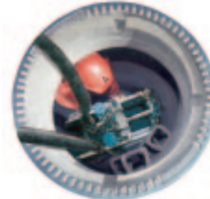
Grundopit - house connection technique Standard version: OD ≤ 110, 50 m Power version: OD ≤ 160, 80 m
