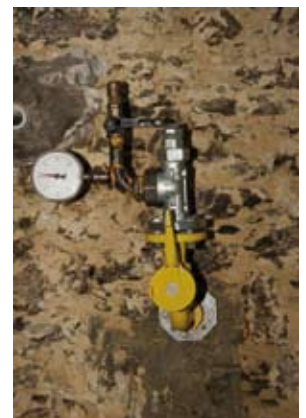
House connection: start directly out of the cellar - tested and recommended by E.ON.
