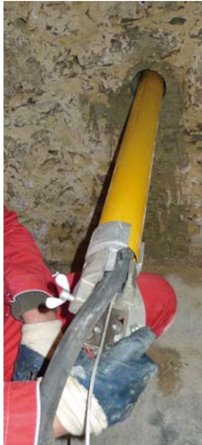
House connection: start directly out of the cellar - tested and recommended by E.ON.
