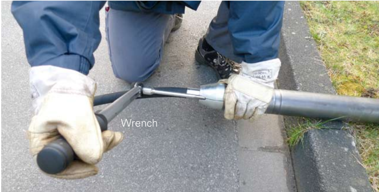
Simple exchange of the reverse cone for a pull sleeve on site.
