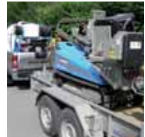
Installation of sewage pressure pipes.
