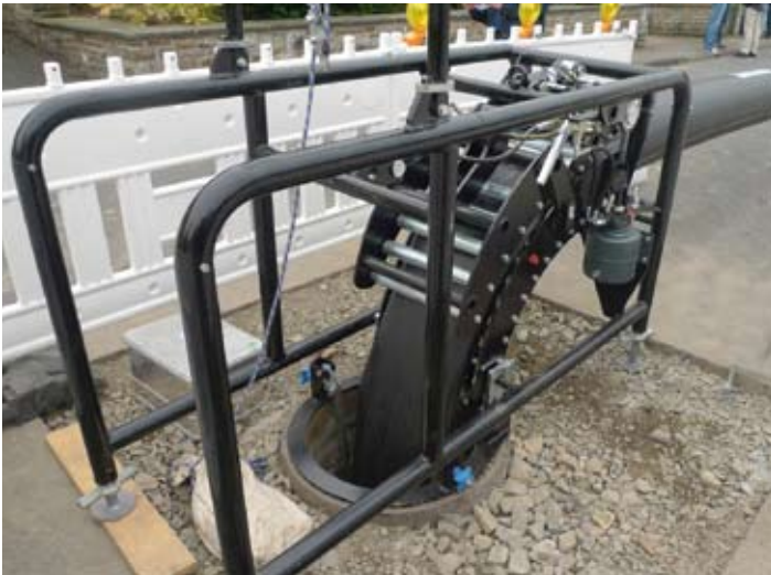
BURSTFORM - Installation of long pipes from manhole to pit.
