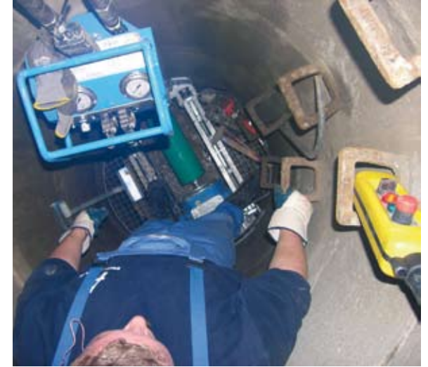
GRUNDOBORE - Auger boring systems.
