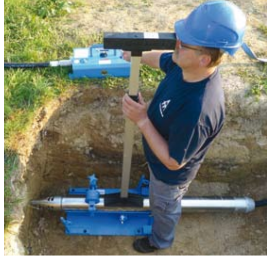
GRNDOMAT soil displacement hammer.
