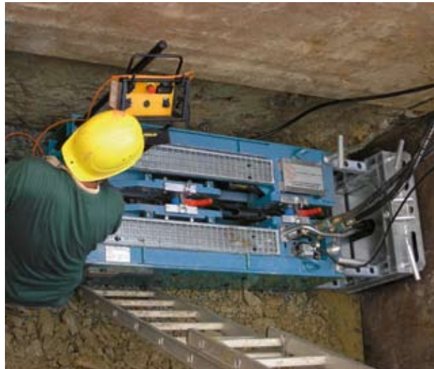
GRUNDOBURST - Static pipe bursting.
