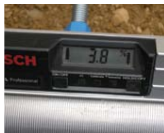
Pilot bore with GRU 95: Adjusting to 3,8 % inclination.
