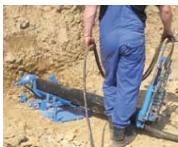
Pushing the SL canal pipes with a hydraulically operated tensiometer.
