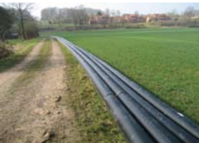
Pipe lengths ready for installation.
