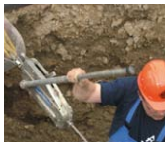
Support by a pulley inside the target pit.
