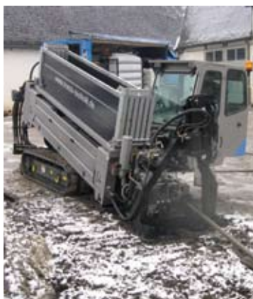
The start of the pipe installation can be steered and checked with a remote control directly from the installation pit.
