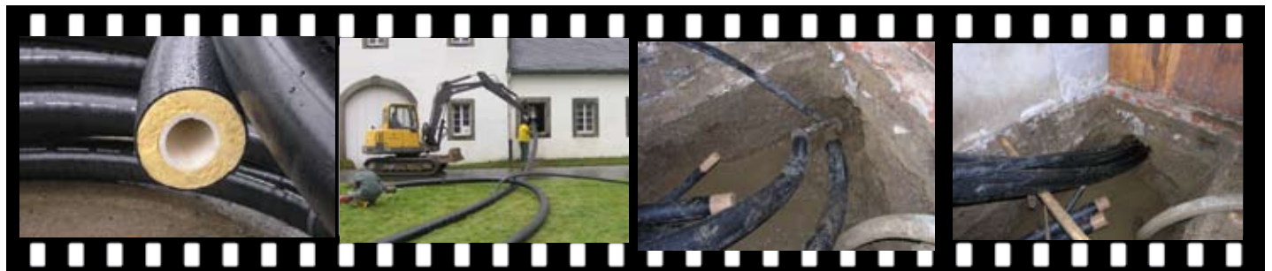
Cross-section of long distance heating pipe.
