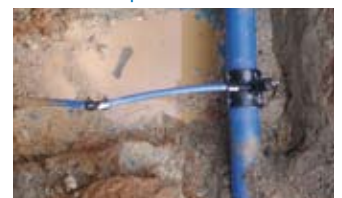
The new endless drinking water pipe PE 100, DA 32 x 3 mm.
