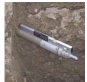
In the target pit: Re-checking the Inclination.
