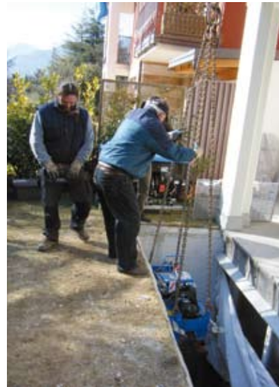
GRUNDOPIT placed into the light shaft with a crane. The picture below shows the power unit TT B 20.
