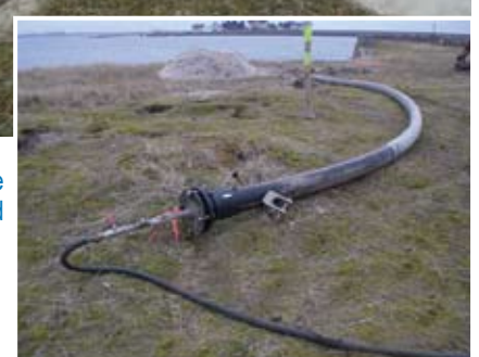
Installation of the empty pipe and cable injection.
