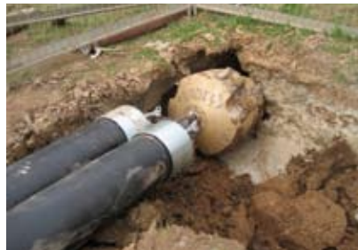
Starting the pulling-in process.
