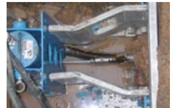
Grundotugger: new pipe arriving in the machine pit.
