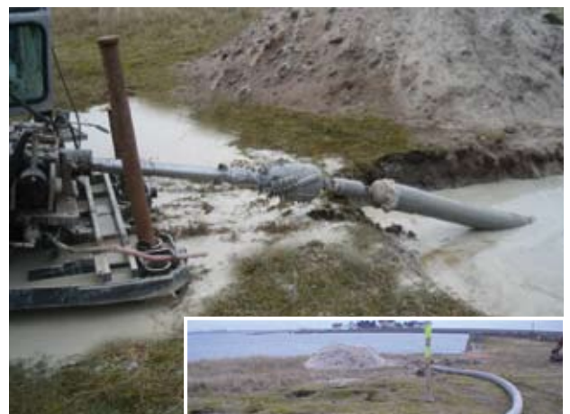
Installation of the empty pipe and cable injection.
