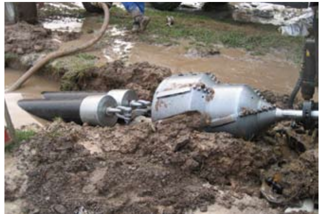
Pipe installation completed.
