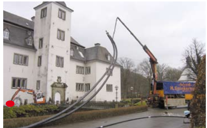
Connection of the pipe length inside the installation pit (red spot).
