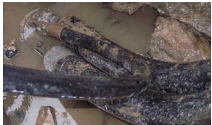
The start of the pipe installation can be steered and checked with a remote control directly from the installation pit.
