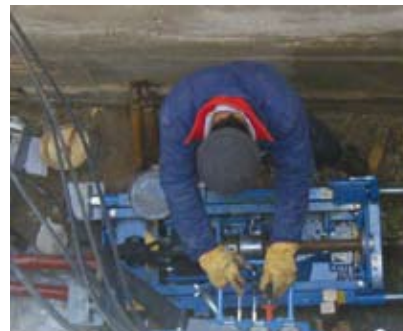
GRUNDOPIT during the pilot bore.
