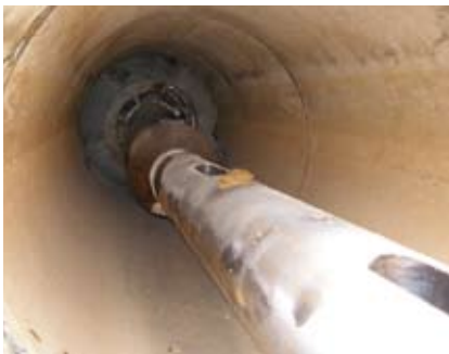
Starting the bursting process and destroying the old pipe.
