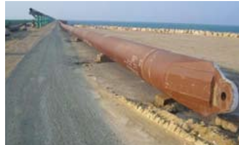
The 800 m oil pipeline ready for installation.
