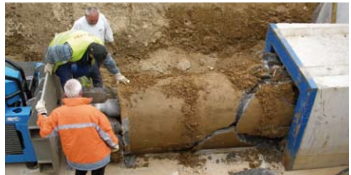
End of the bursting process and arrival inside the machine pit.
