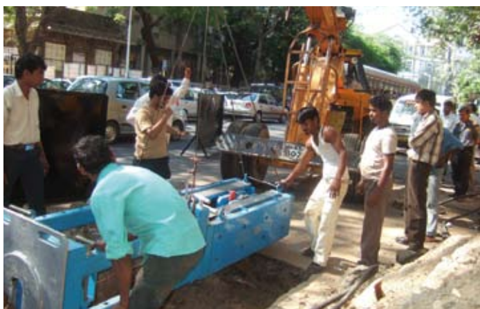
Installation of the GRUNDOBURST in the working pit.
