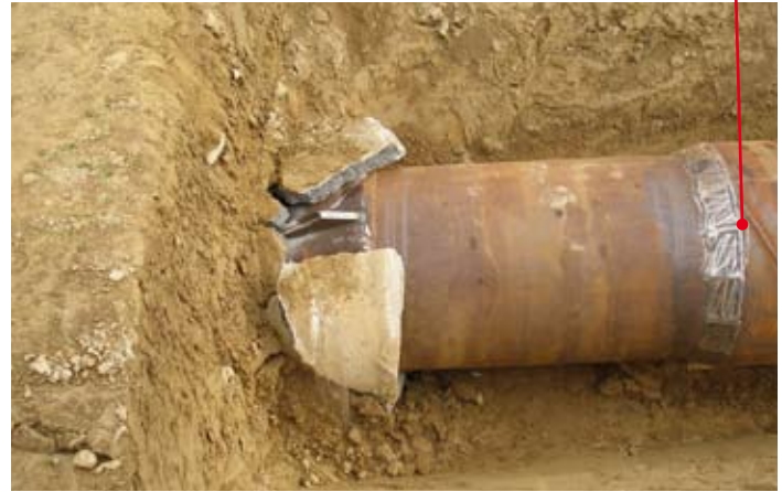
Starting the bursting process and destroying the old pipe.
