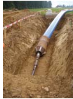
The pipe length shortly before starting the installation with two-step expanding process.
