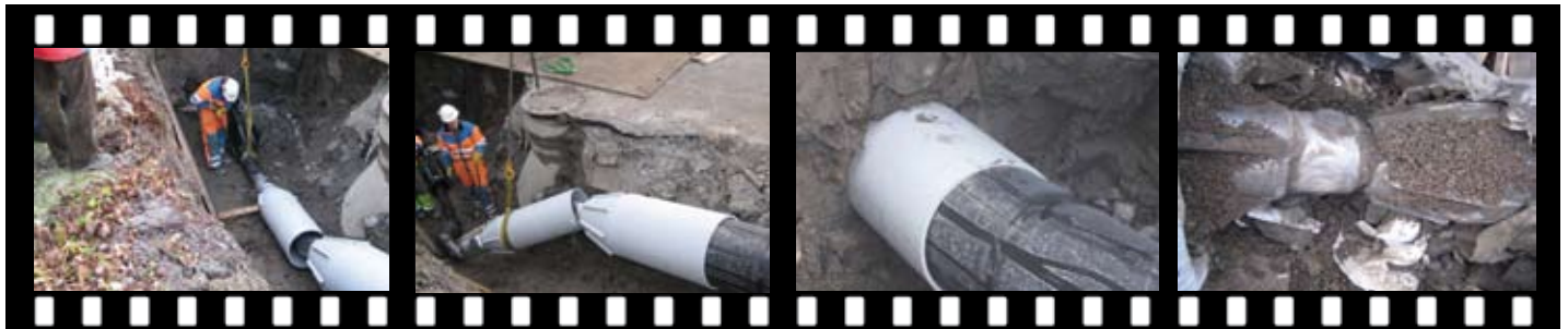
GRUNDOBURST 2500 G during pipe installation.
