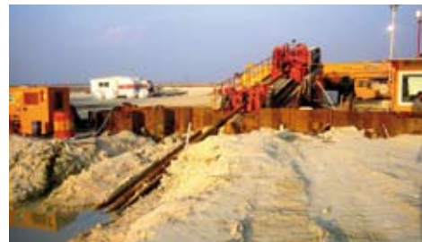
HDD-bore rig 250 t on the mainland.
