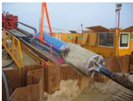
Adapter to HDD-Rig with Taurus rammer and suitable cone.
