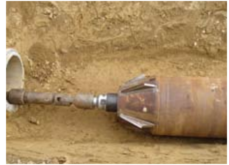
The pipe length shortly before starting the installation with two-step expanding process.
