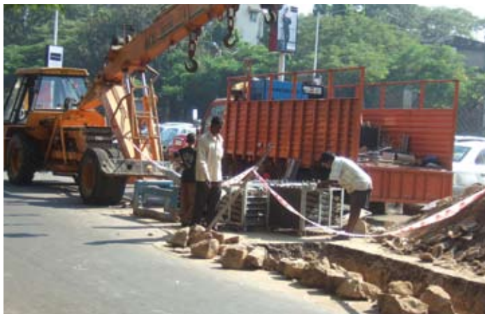
Overview of the GRUNDOBURST jobsite in Mumbai.
