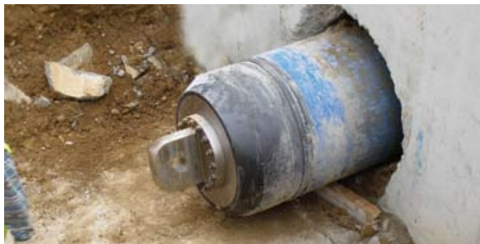
The new pipe with pulling eye after installation.
