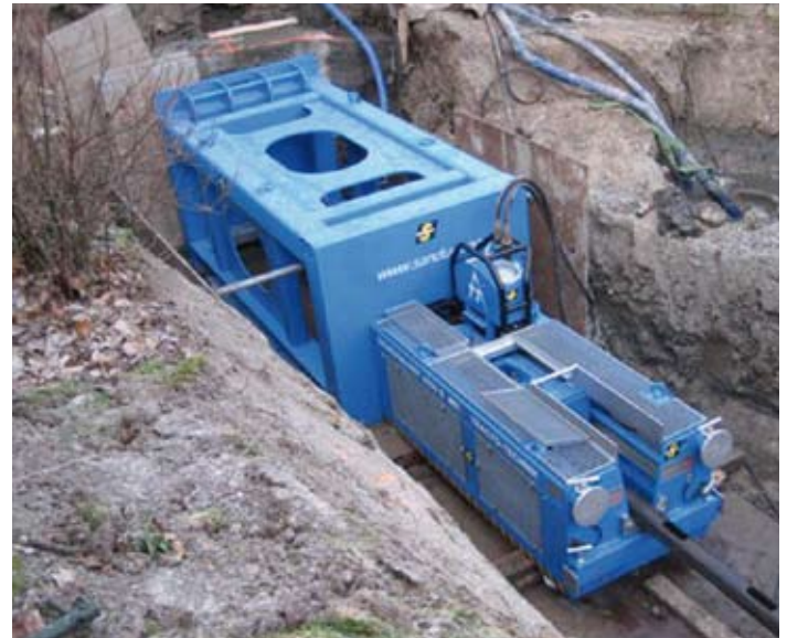
GRUNDOBURST 2500 G during pipe installation.
