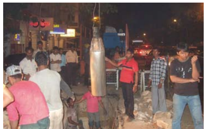
Retrieval of the expander from the target pit.
