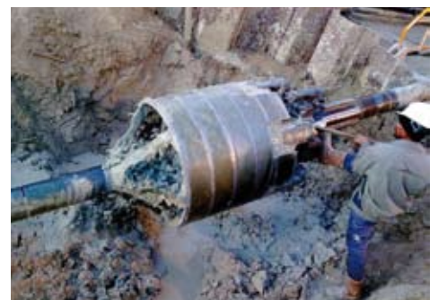
After freeing the drill rods, it was possible to retrieve the backreamer.
