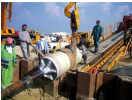
Adapter to HDD rig with flanged on HDD drill rods.
