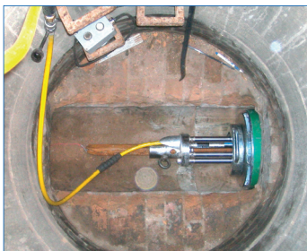
View inside the canal manhole with Burstfix.
